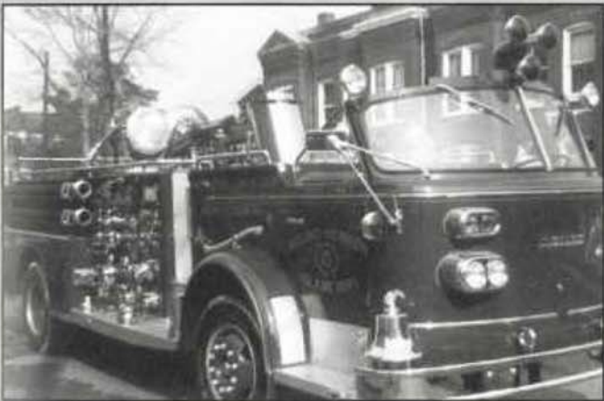
Mt. Vernon purchased a unique engine powered by a Boeing Turbine engine. Complete with a large exhaust stack, this 1962 American LaFrance was only one of four produced with the unique motor. Called the "Turbo Chief", the four trucks proved to be unpopular. Mt. Vernon's American LaFrance was later changed to a gasoline engine. (John Floyd photo).
