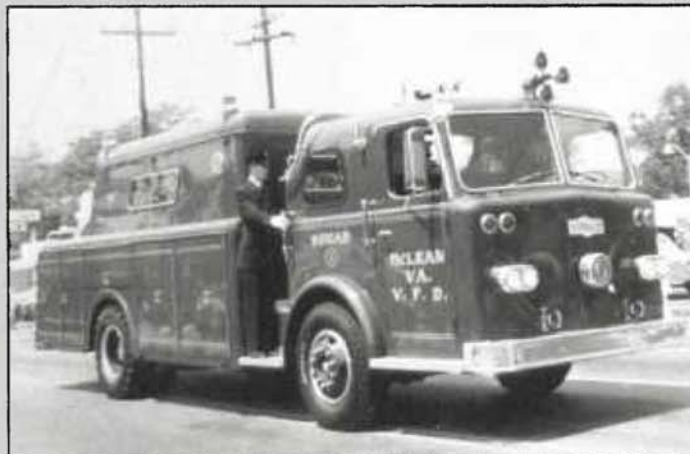
McLean purchased an unusual rescue squad in 1964. The cab was a Pirsch, and Gerstenslager built the body. This truck also had a 200 gpm pump and carried 200 gallons of water. (John Floyd photo).
