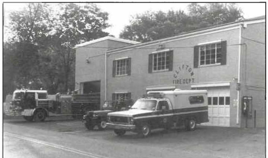
Clifton Fire Station before it was rebuilt featuring an Imperial Pumper, Jeep brush unit and an ambulance.
